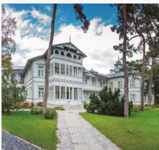
Gurewicz Spa Resort. Hotel- Restaurant - Spa. Otwock, Polen. PACi, VRF og Styling.
